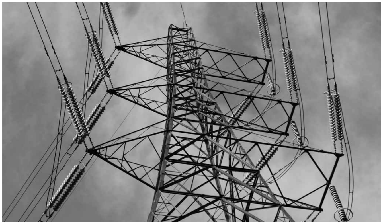
The 20 MW waste heat recovery based power plant has got registration under UNFCCC for carbon credits. We also envisage setting up a char fuelled bed captive (CFBC) power plant.
